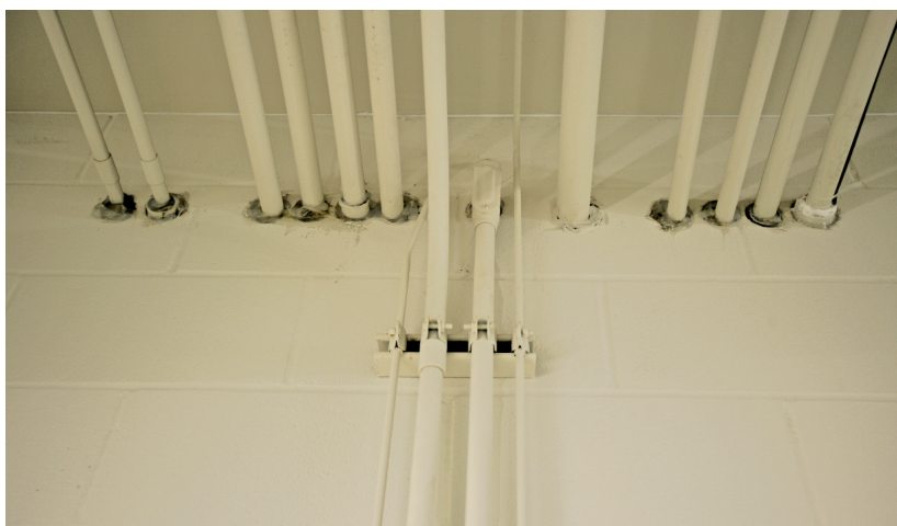
FIGURE 18. Caulking around Service Intrusions*
